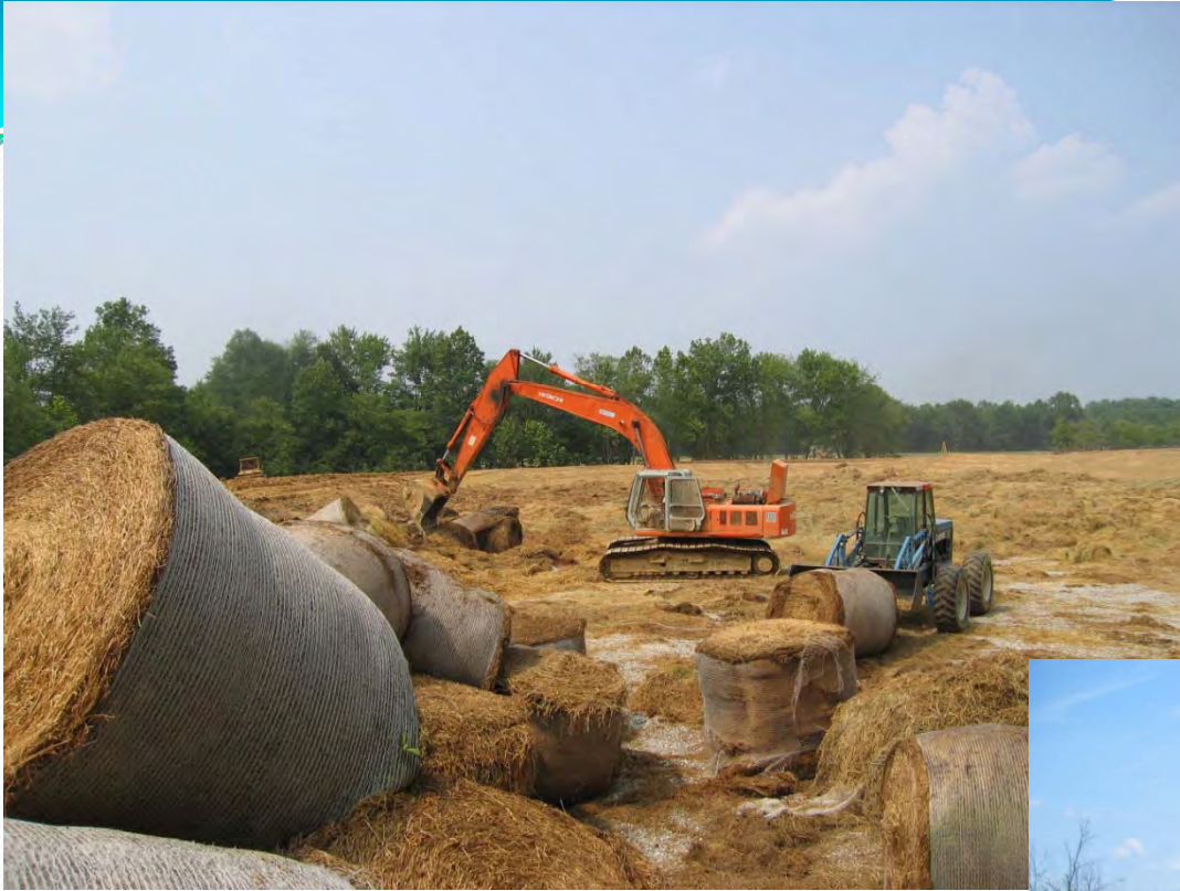
Placement of the Compost Layer: West VFP.
